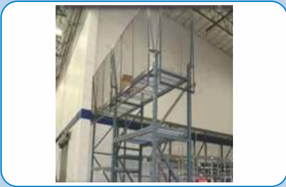
PALLET RACK FALL PROTECTOR
